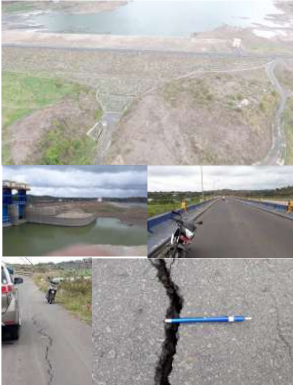
Figure 8 the inspection on hydromechanics of Pandanduri Dam
